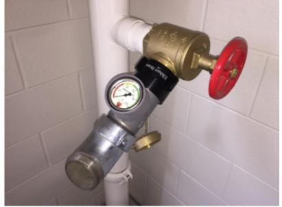
The above picture shows the hook up order on the standpipe. The inline pressure gauge goes on first. The ideal pressure we are looking for at the standpipe is 65psi. It will still work quite well at lower psi's, which is a reason we moved to  $2\frac{1}{2}$  hose with a smoothbore.
